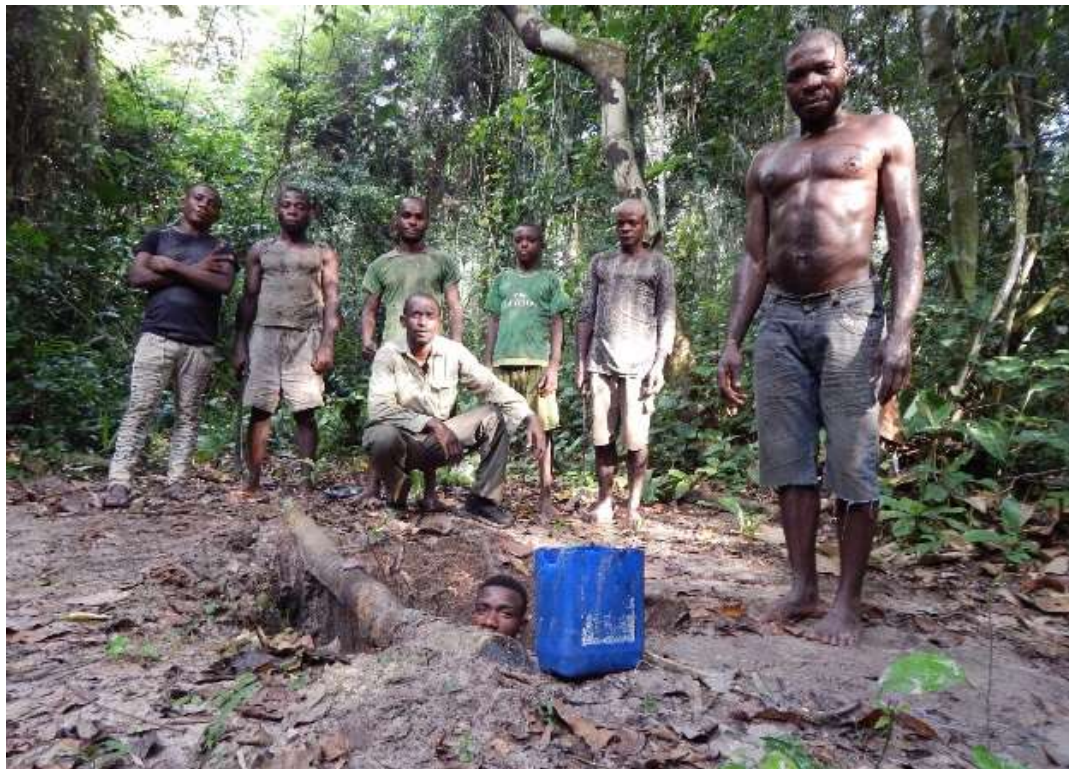
Another group of hunters is digging the well for water near the camp
