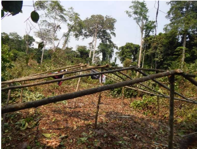
Constructing a temporary house
